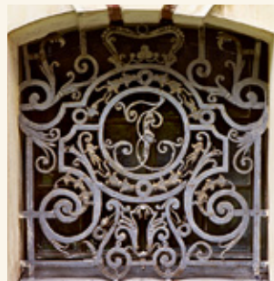
Lattices of the Vault's window with the monogram of Duke Ernst Johann
